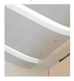
of vaulted semi-circular GRG panels inlaid with rebated features including the installation of dummy columns and wall linings. The main sales area ceiling comprised 4400m² of a metal concealed Burgess system together with 1100 linear metres of integrated trough lighting.
